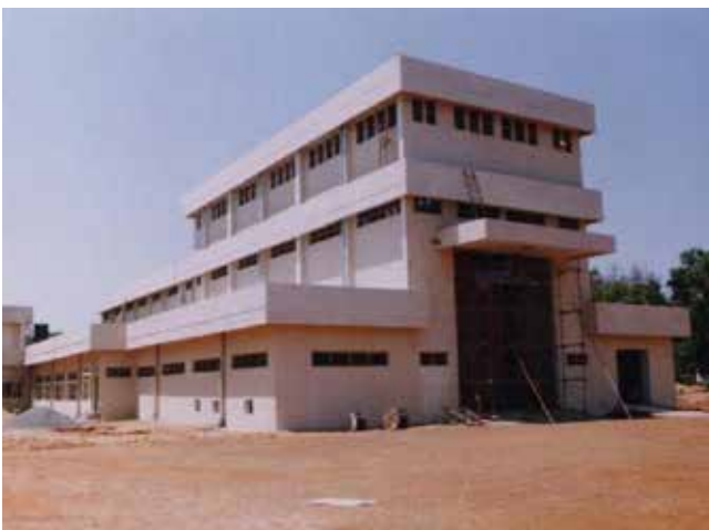
Vehicle Integration facility
